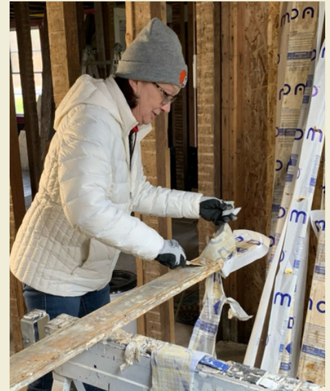
Volunteer and Museum Development Committee Member Cathy Berlo works tediously stripping away layers of paint from an original piece of trim.
